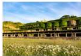
KITAZAWA FLOTATION PLANT
