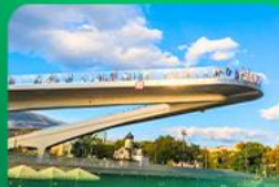
Floating Bridge Moscow
